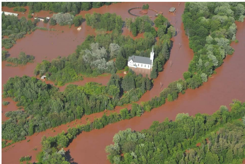
Figure 3-8: Flooding from the Bad River in Old Odanah, Ashland County. Photo from Civil Air Patrol flight, July 12, 2016.
