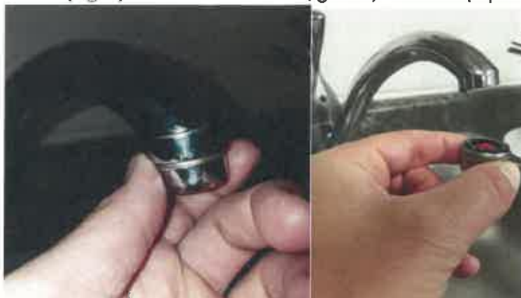
Figure 3. This is an example of a metal, indoor faucet located after the pressure tank and water treatment system (with aerator being removed).
