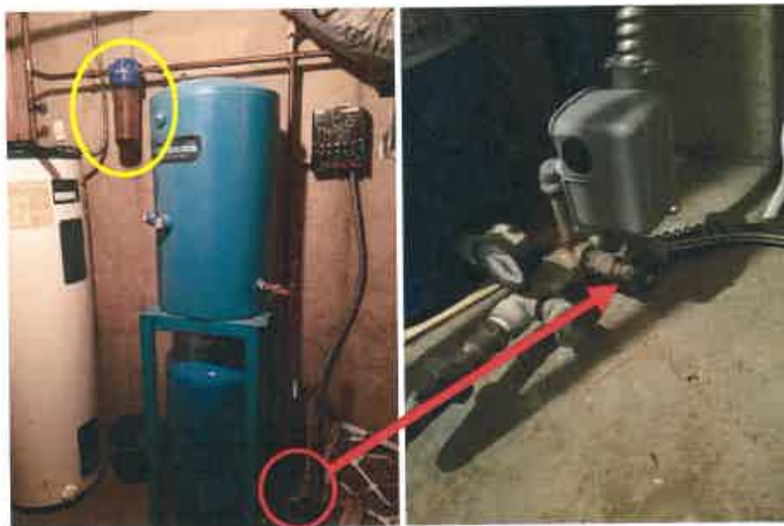
Figure 2. Photograph of a sample faucet located after the pressure tank (circled in red/red arrow) but prior to a carbon filter (circled in yellow).
